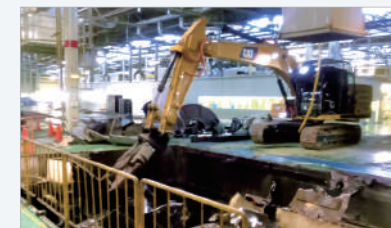
Dismantling of Painting Facilities
